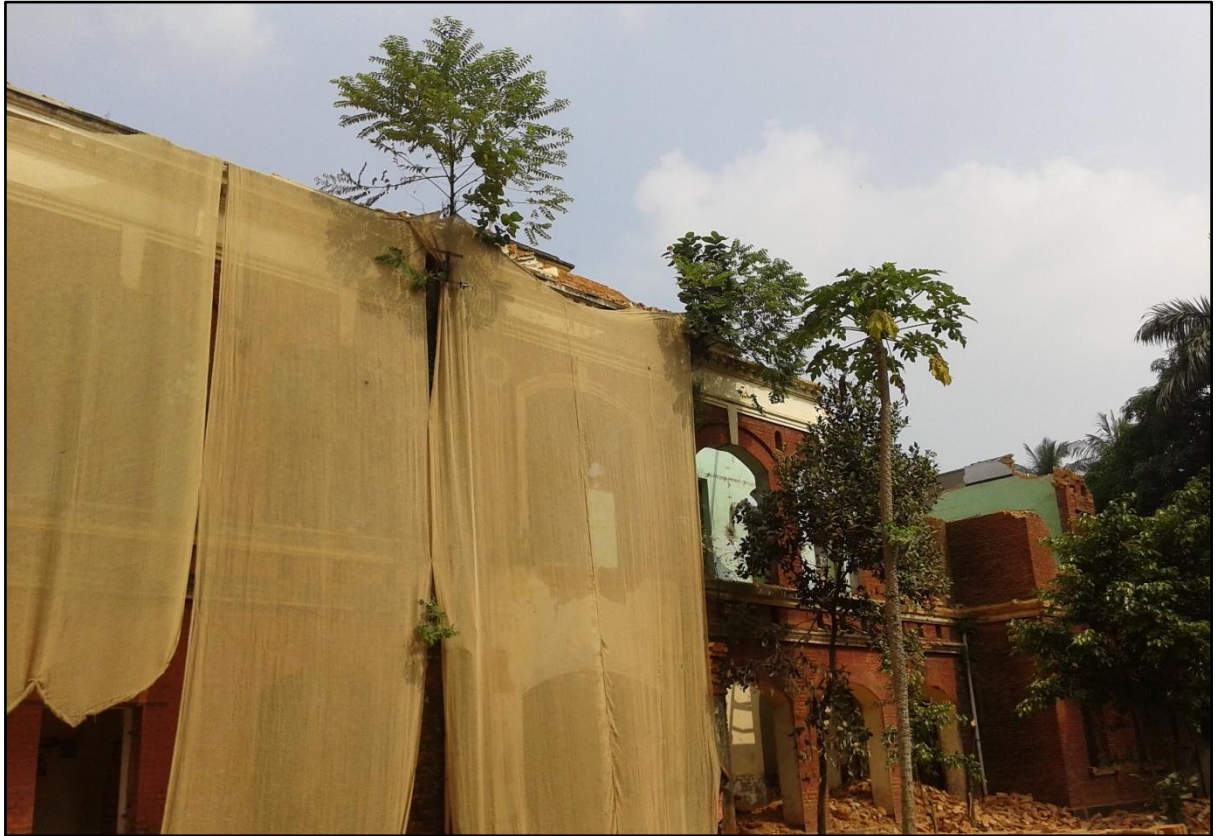
Figure 19: Partially demolished heritage site and century-old laboratory building in Khamarbari.
